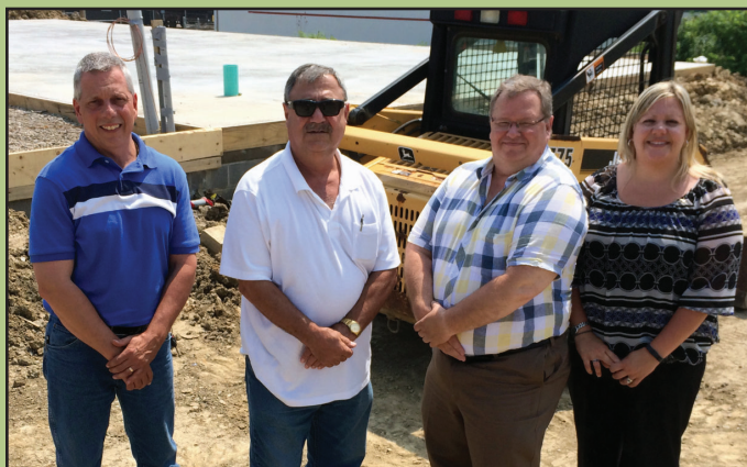
O.H.I. Ice Cream Distributors, Inc. marks the first business to take part in the WCCED's Main Street Loan Program. Pictured are Tim Jankowski and David Minor of O.H.I. with Dan Reitz and April Cacia of WCCED at the construction site of O.H.I.'s new facility.
